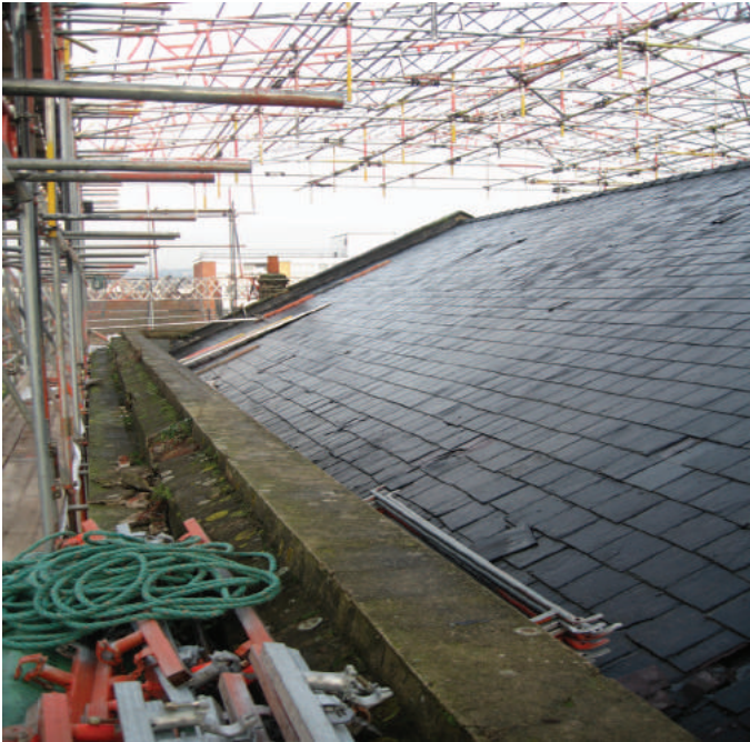
New roof installation on completion
