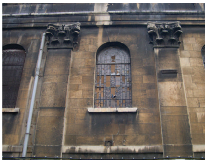
Detail of exterior facade in Nov 2005
