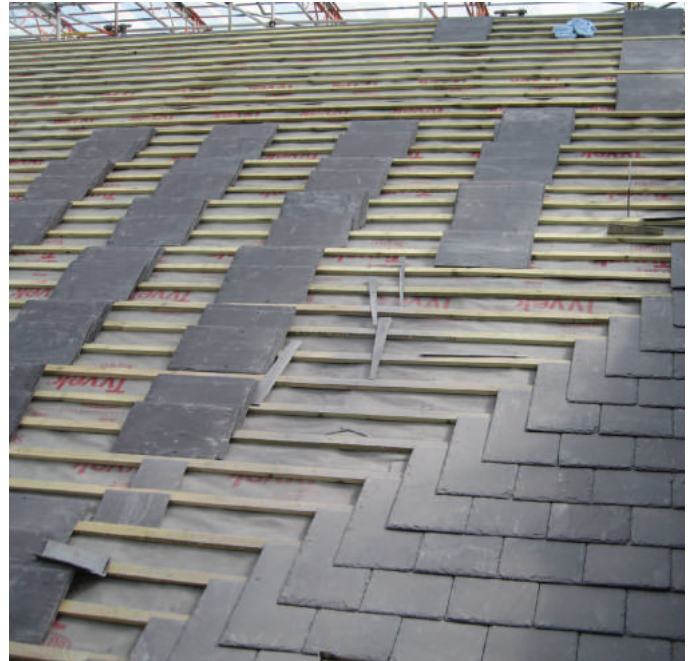
Installing new UK sourced roofing slate
