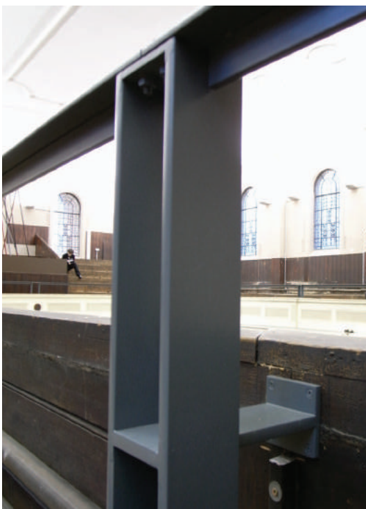
New balustrade installed to support the existing timber balustrading & satisfy the regulations
