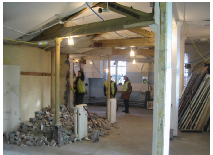
Removing the more recent additions to reveal the original architectural features
