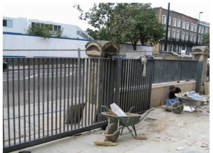
Installation of reclaimed sandstone paving slabs from sustainable source
