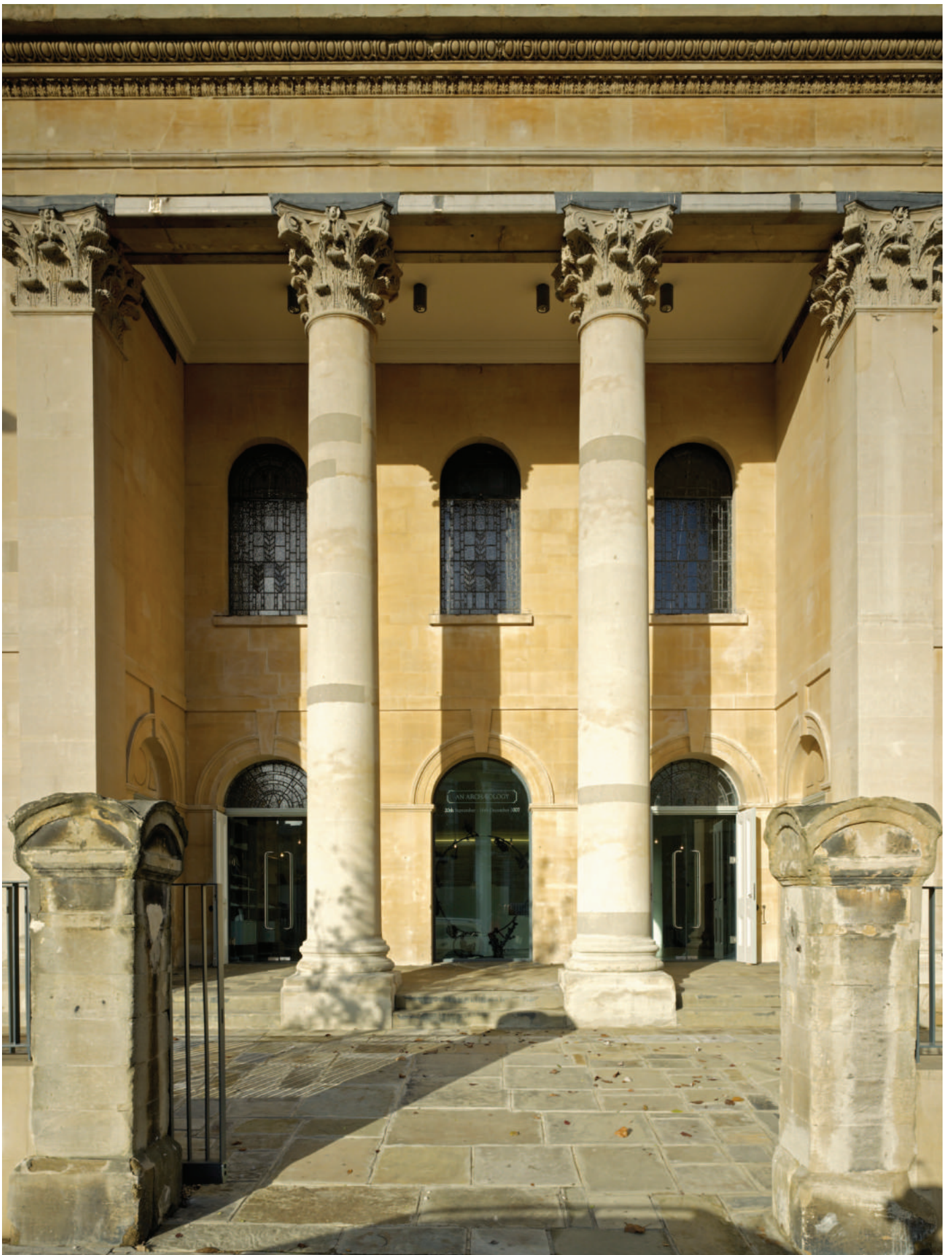
The refurbished entrance portal and landscaping
