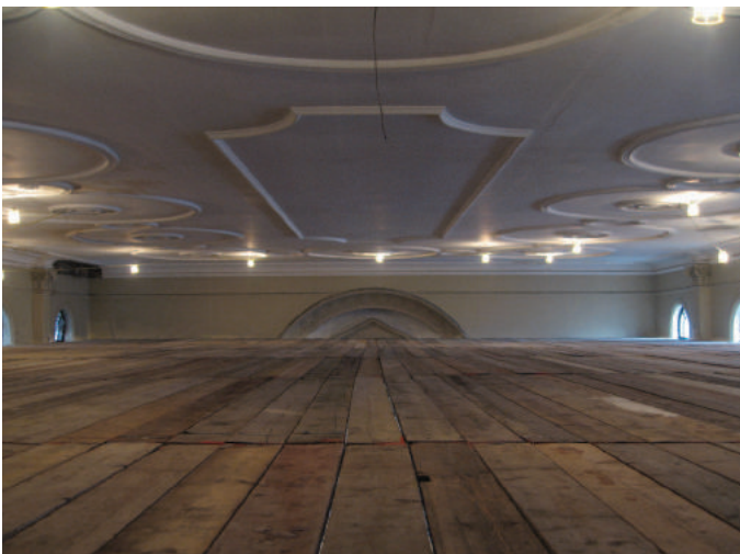
Combating the extensive dry rot & repair of the original ceiling plasterwork
